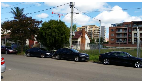
Figure 5- No.11 and 13 Goulburn Street, weatherboard dwellings in deteriorating condition
